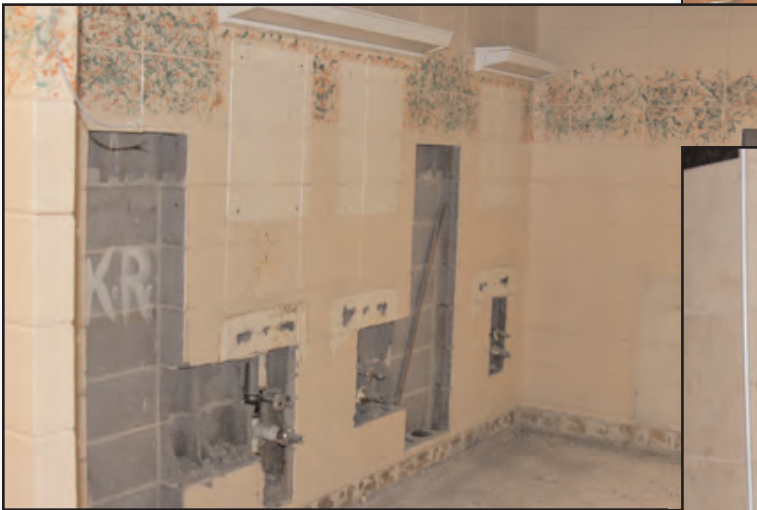
The Men's Restroom before...
